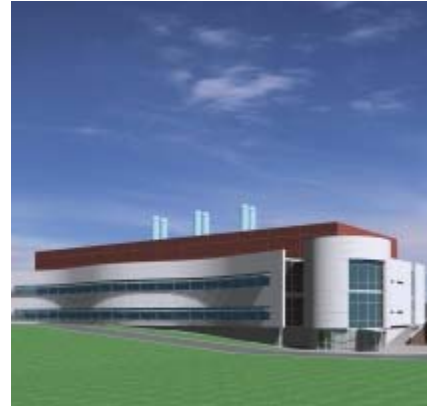
The 72,000-square-foot, $53 million facility will be the latest addition to Colorado State's Infectious Disease Research Center.
